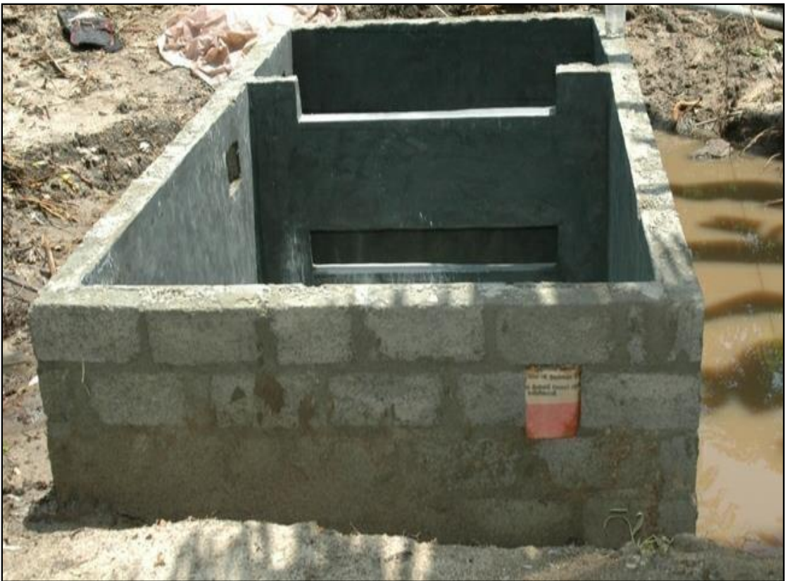
Fig. 6.4: Storm water and Waste water collection tank
